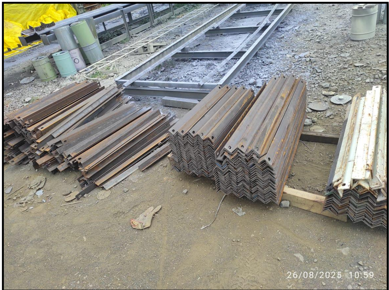
Figure 32: Stacked Steel Angles and Fabricated Members Ready for Assembly
