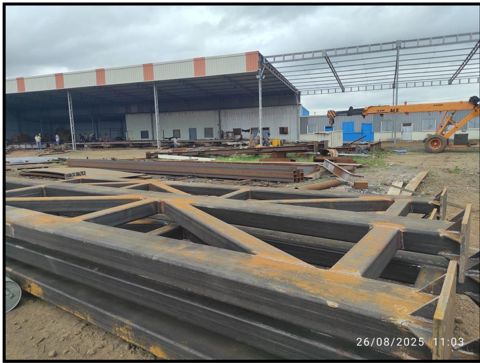
Figure 11: Structural fabrication yard (steel components for industrial sheds).
