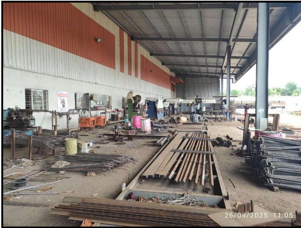
Figure 33: Steel Fabrication Workshop with Cutting and Bending Operations
