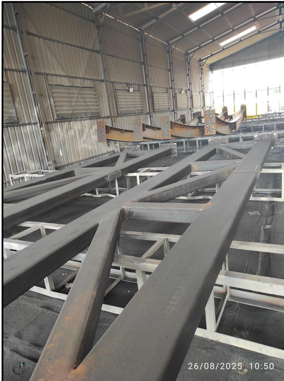
Figure 29: Steel Truss Fabrication and Assembly
